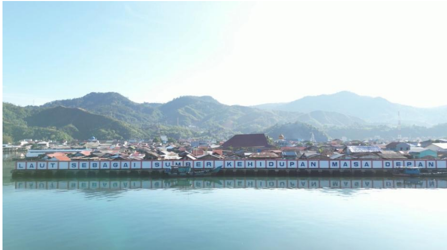
Gambar 5.4. Foto Retaining Wall
