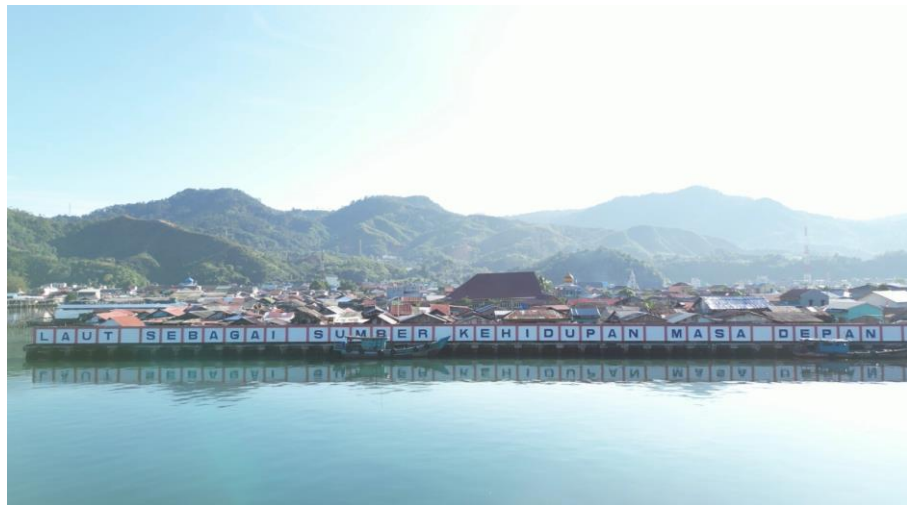
Gambar 5.4. Foto Retaining Wall
